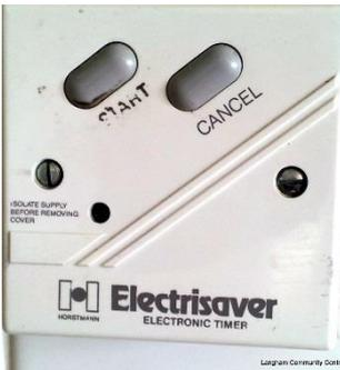
This switch is in the kitchen by the hatch. Press *Start* to heat the hot water in the kitchen and main hall toilets. This will stay on for 2 hours unless you press *Cancel*.
